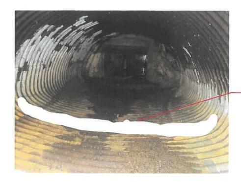
BOTTOM OF CULVERT IS CORRODED- PAVE INVERT WITH CONCRETE
